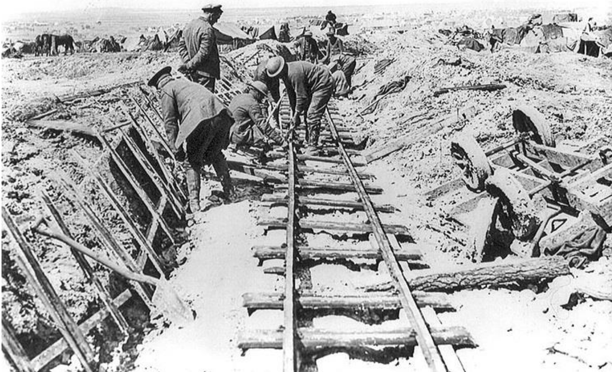
Canadian Railway Troops repairing narrow-gauge track on the Western Front c1917. (Photo courtesy of Library & Archives Canada)
