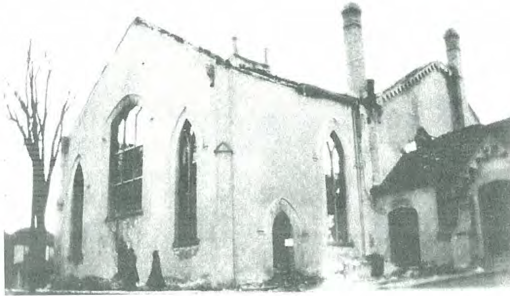
Plate 3: Photograph from morning after the fire showing rear of church (Miller 1992)
