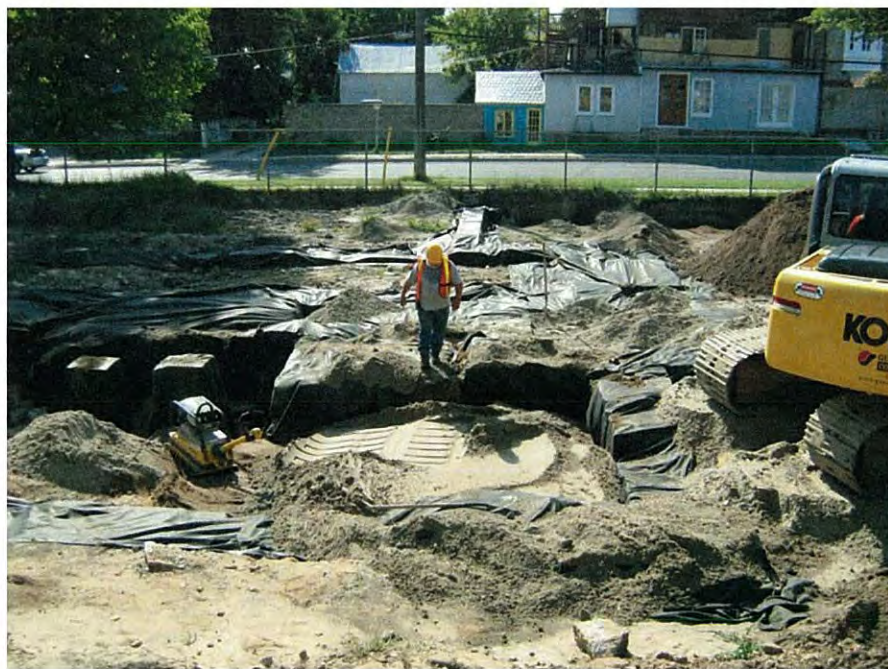
Plate 28: Covering the wall of 1832/33 church with geotextile
