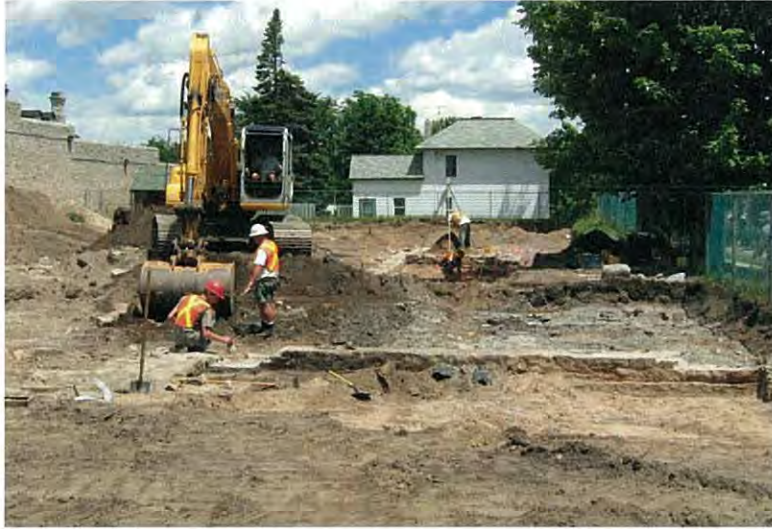
Plate 21: Mechanical stripping and hand excavation to expose the church walls
