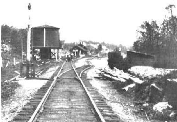
**Perth built water tank installed at Ardentale, Ontario**
