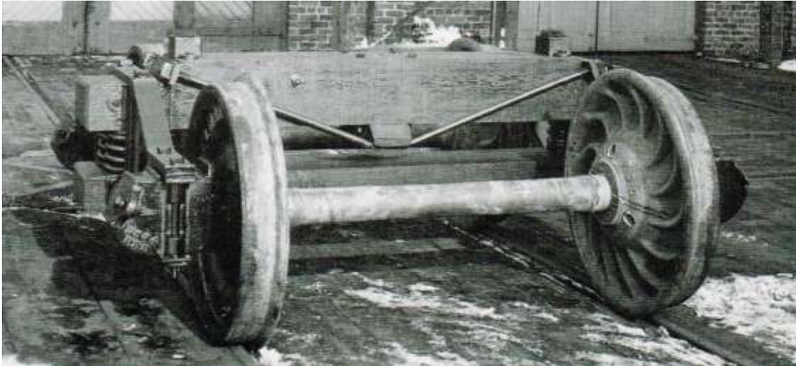
*Example of an Arch Bar Wood Beam Truck of the type manufactured at Perth<sup>19</sup>*
